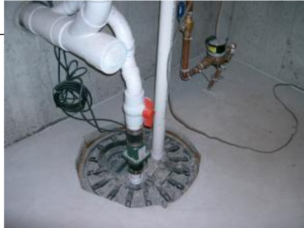
Sump pumps should have tight fitting cover
