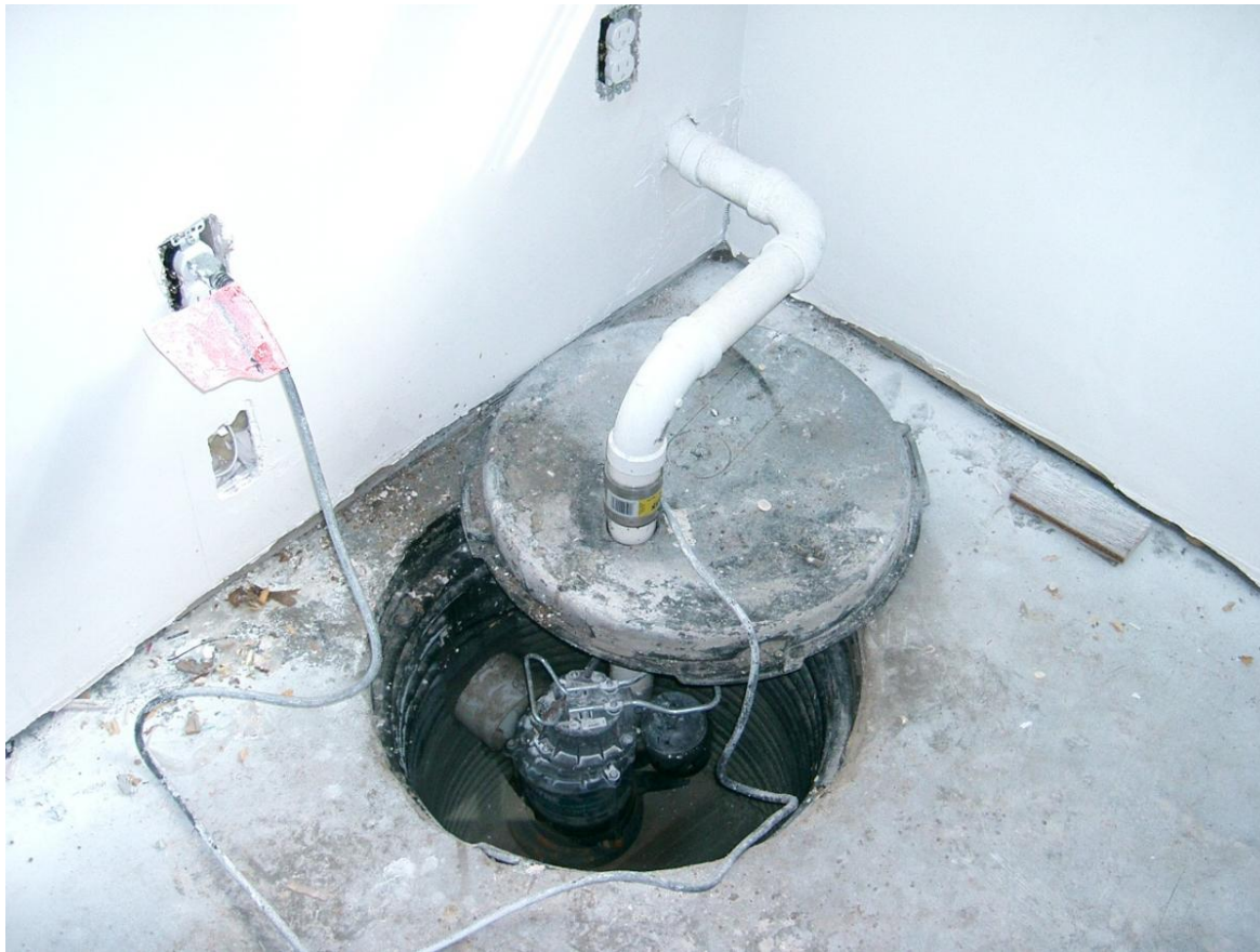
Figure 5. Install the sump pump cover. (Source: Building Science Corporation ( https://basc.pnnl.gov/library/building-science-corporation-bsc .)
