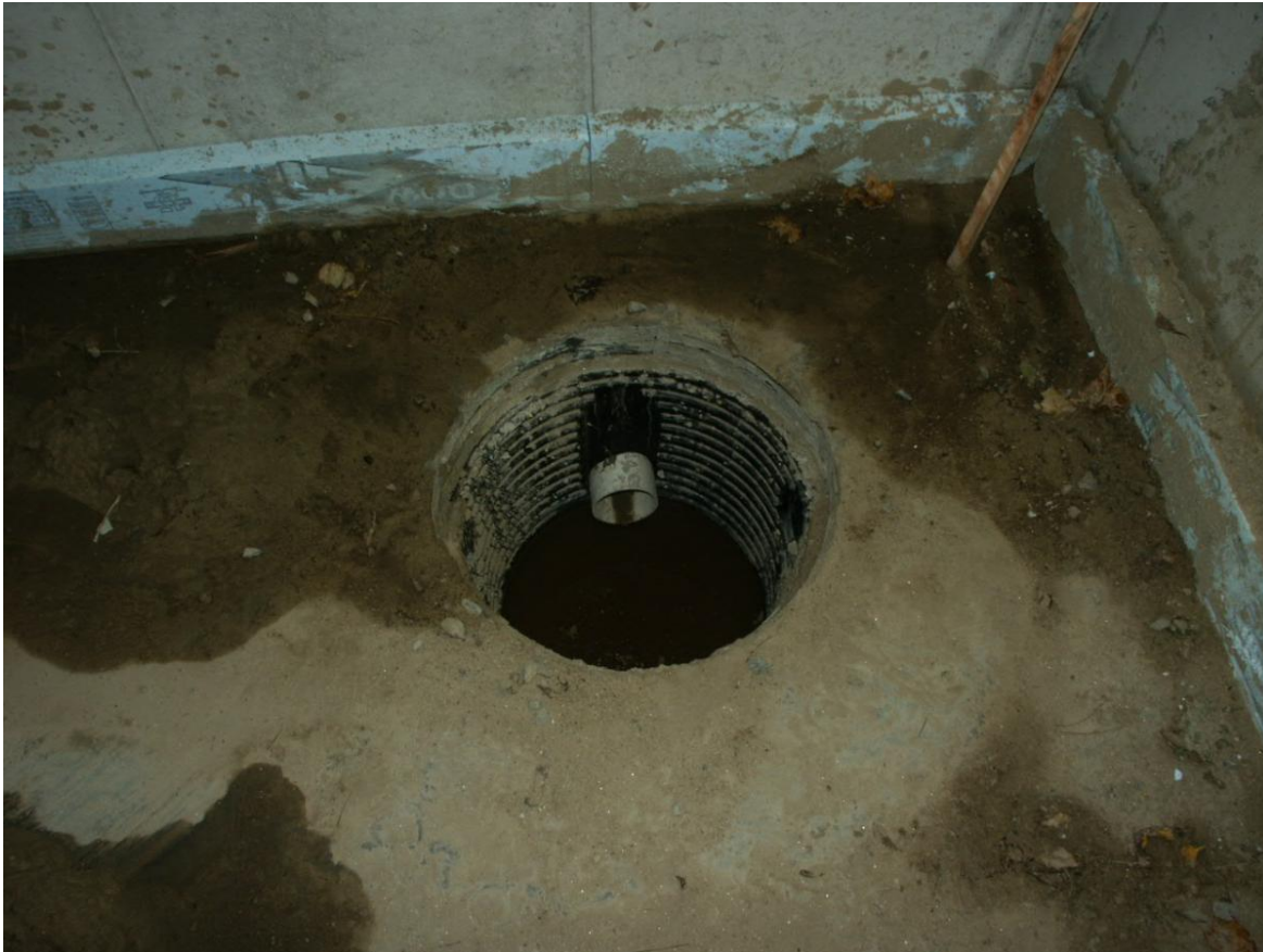
Figure 3. Install the sump pit liner. (Source: Building Science Corporation (https://basc.pnnl.gov/library/building-science-corporation-bsc) .)
